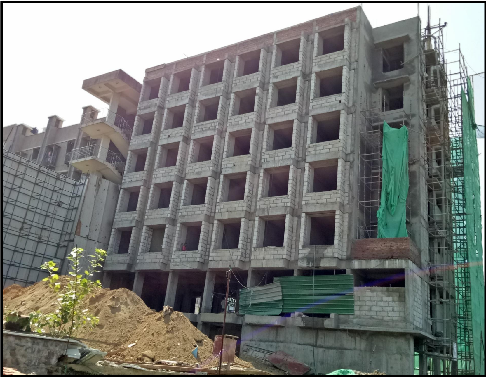
Extension Hostel Blocks G1
