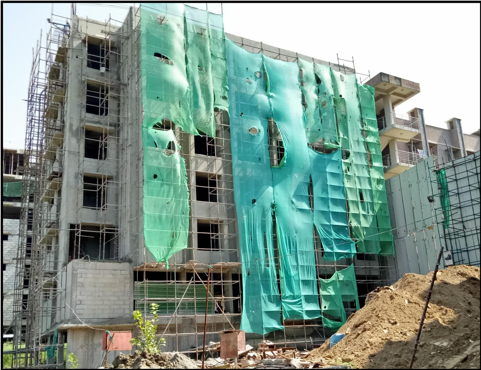
Extension Hostel Blocks G2
