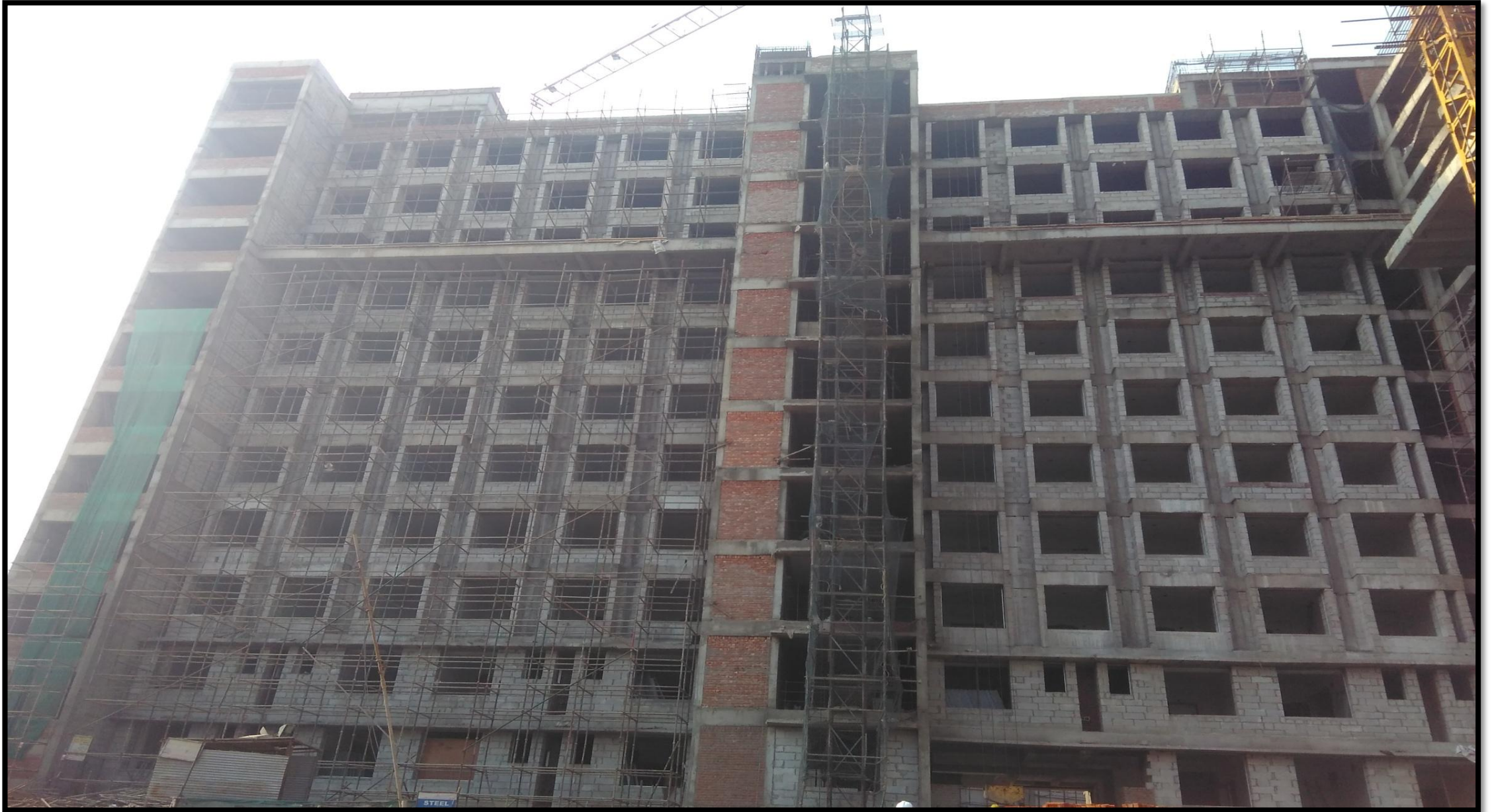
Hostel Blocks H1
