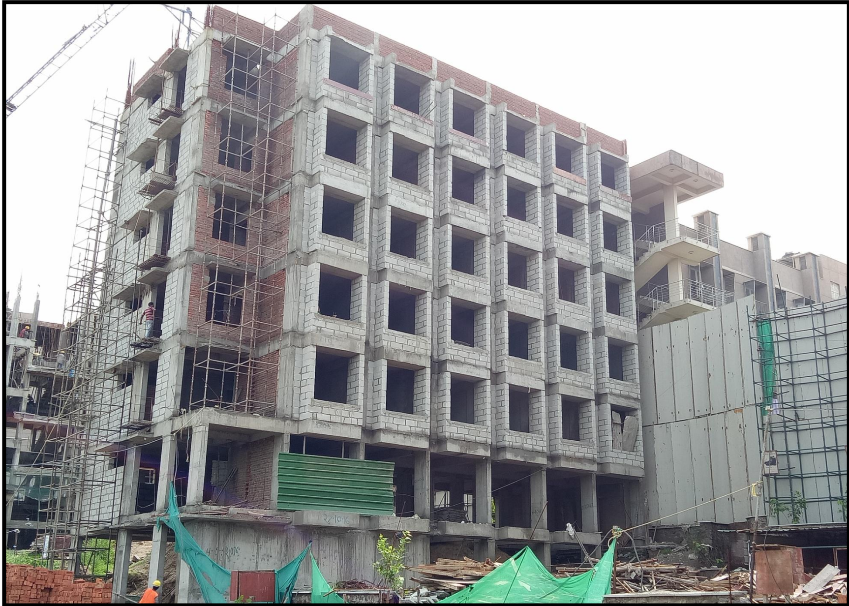
Extension Hostel Block G2
