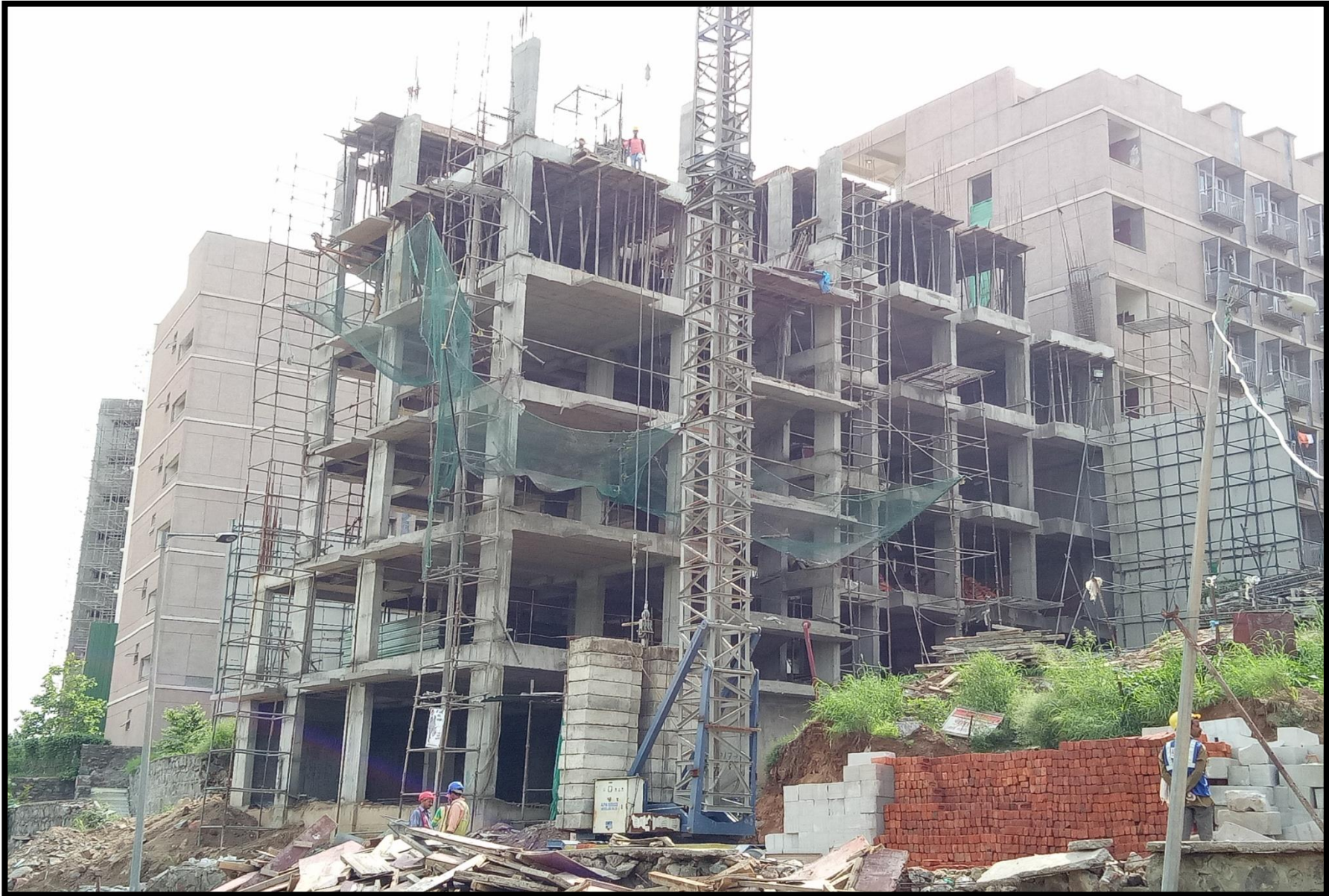
Extension Hostel Block B1
