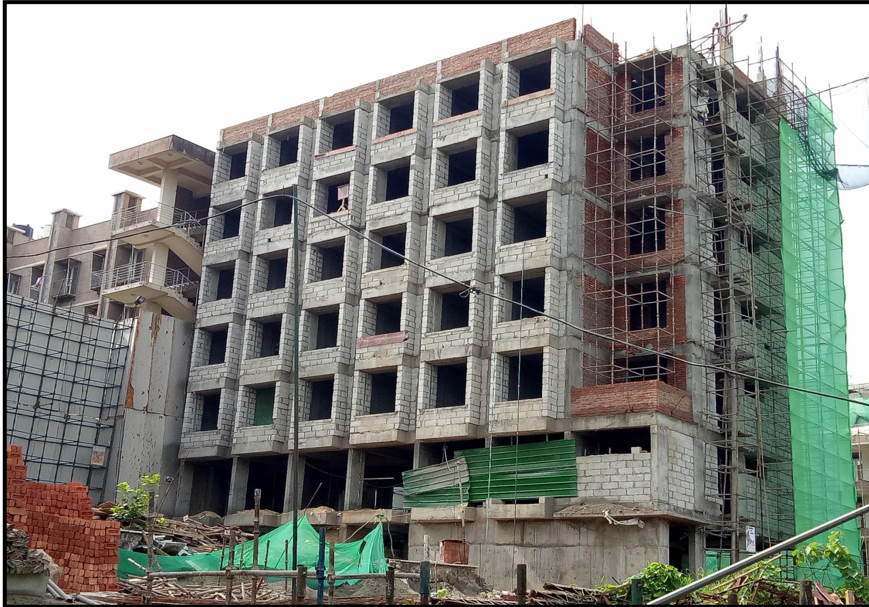
Extension Hostel Block G1
