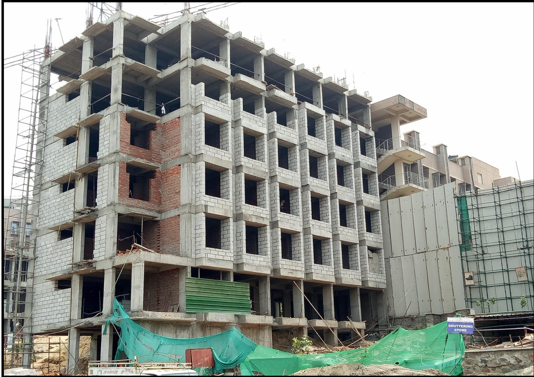
Extension Hostel Blocks G2
