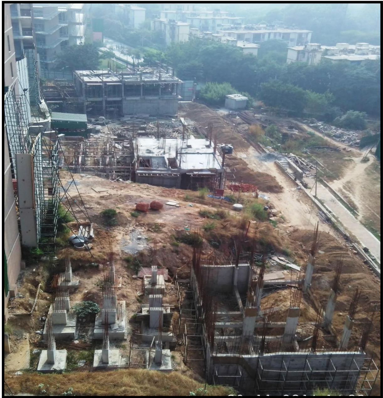
Extension Hostel Blocks G1, G2 & B1
